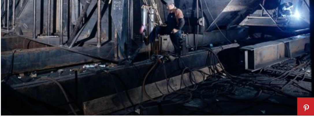
Constructing the crawler-transporters in Marion, Ohio, 1964.
